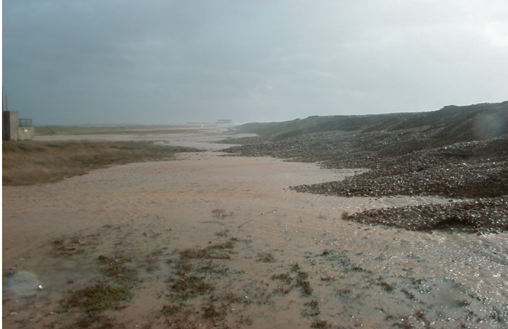
Medmerry, by sluice, looking East, November 2005 Copyright Chichester District Council
