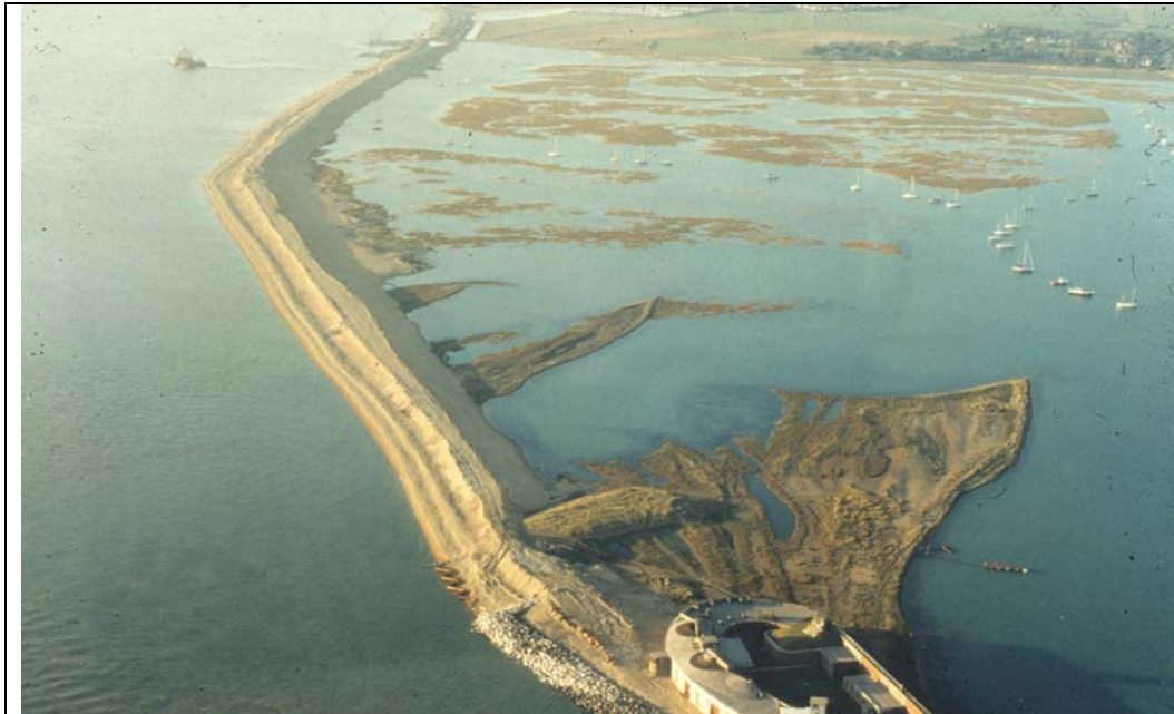
Hurst Spit Stabilisation Scheme 1996-1997 Copyright David Bowie Photography
