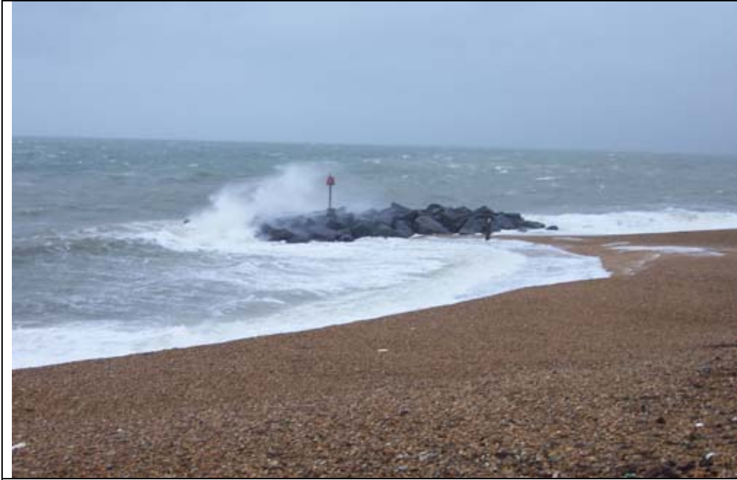
Hurst Spit rock breakwater Copyright New Forest District Council
