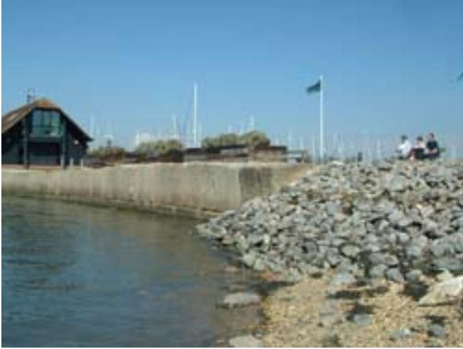
Rock sea defences at marina, August 2005 Copyright Chichester Harbour Conservancy
