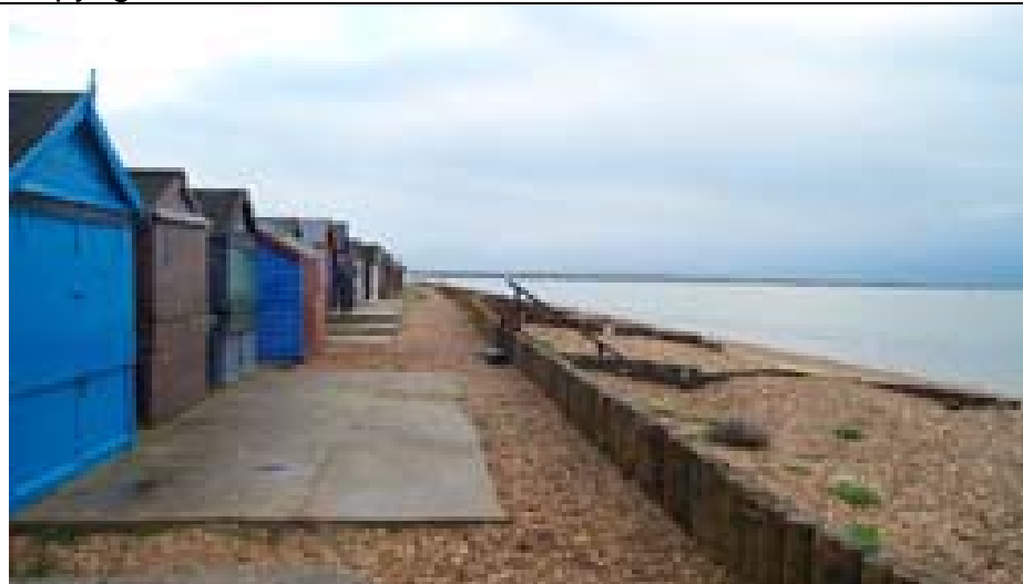
Calshot Spit, timber revetment and groynes October 2008 Copyright New Forest District Council
