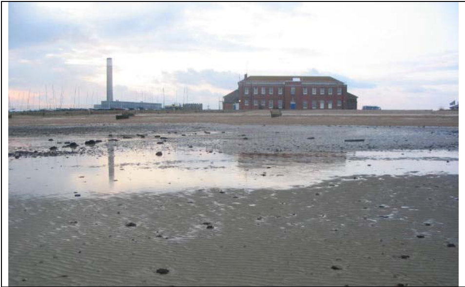
Calshot Spit Activity Centre accommodation with Fawley Power Station in background February 2005 Copyright New Forest District Council
